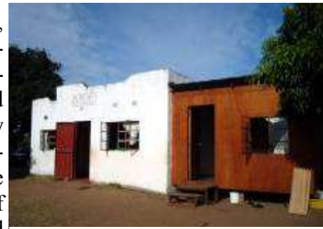
School building and kitchen store room
